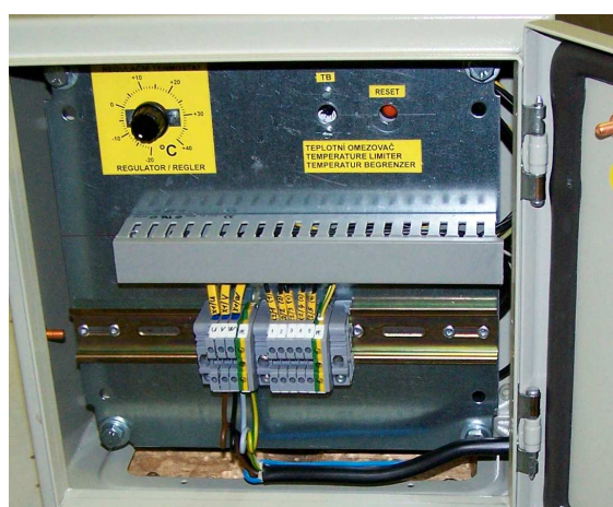
Heating element terminals
