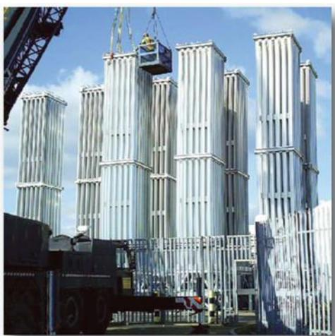
Ambient Vaporizers are intended to evaporate the liquid gas. The Chart-Ferox company is producer of the wide range of the high-pressure ambient vaporizers.
